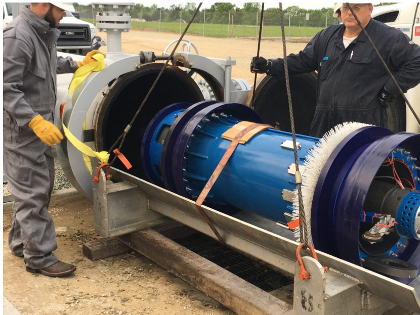
A PIG Being Inserted Into a Pipeline
